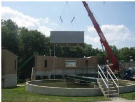
NEW SAND FILTER UNITS BEING INSTALLED
