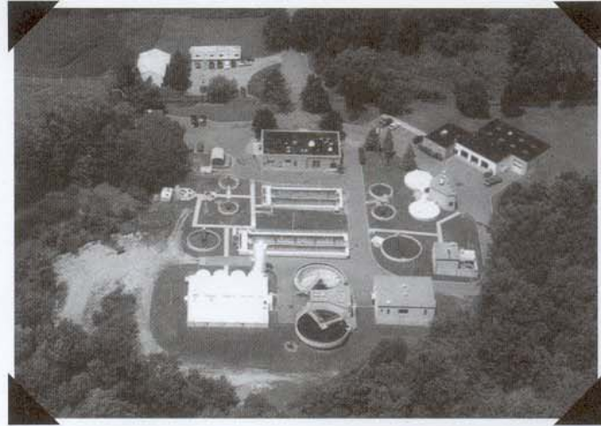
Aerial Photograph of PLBMUA
